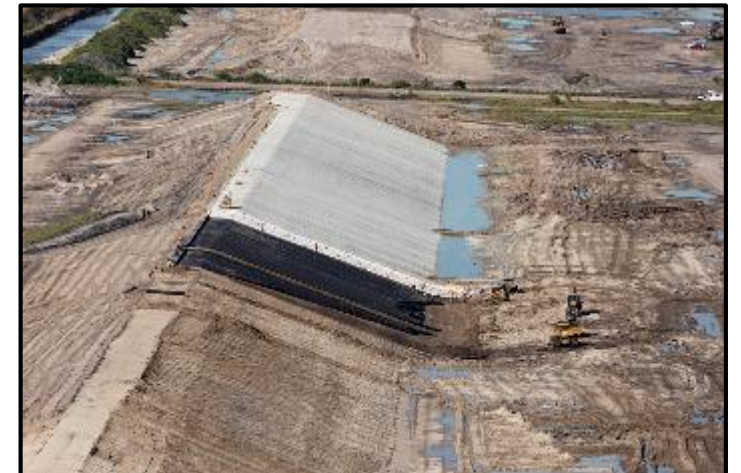
C-44 Reservoir Soil Cement Placement
