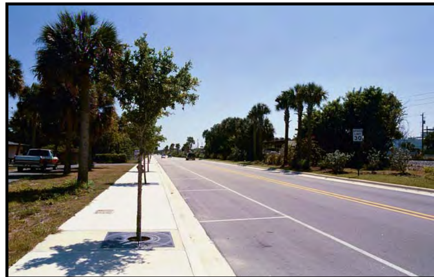
Pineapple Avenue Roadway Improvements
