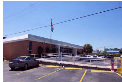
Re-use Of Existing Library Facility
