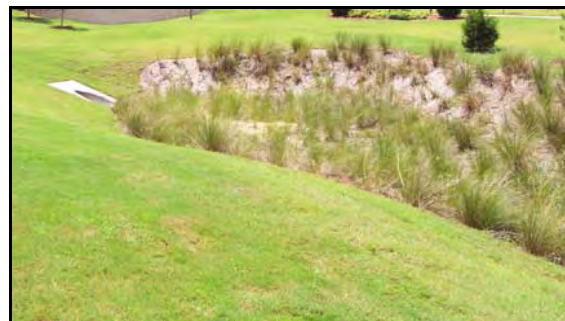
Detention and Drainage Facilities
