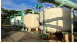
Rehabilitation of four iron treatment filters at the Tropical Farms Water Treatment Plant. Iron treatment filter # 4 will be rehabilitated in FY24 and iron treatment filters #1 - 3 will be rehabilitated in FY30.
