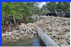
During Hurricane Irma, over 50-acres of primarily red mangrove habitat was lost in the JBI due to high water levels and poor water circulation. In response, the county has secured funding to improve water flow in and out of the impoundment by installing four (4) new culvert connections (drainpipes) to the Indian River Lagoon and dredging the existing channels.
