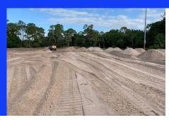
Considering future conditions, the Parks and Recreation Department added 3,461.44 tons of fill to elevate the grade of the Justin Wilson Ball Field to improve drainage. High water table and increased precipitation caused frequent flooding of the park.
