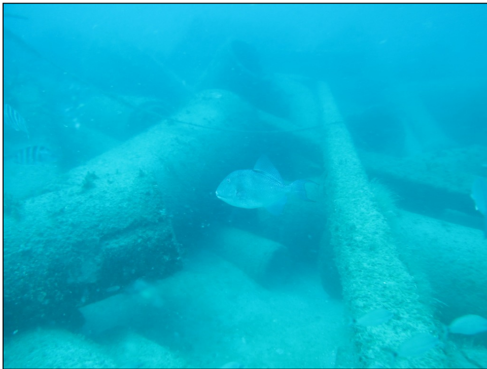
Photograph 1. No obvious damaged, exposed, or corroded rebar was observed on the concrete culverts and poles at South County Artificial Reef Site 15.
