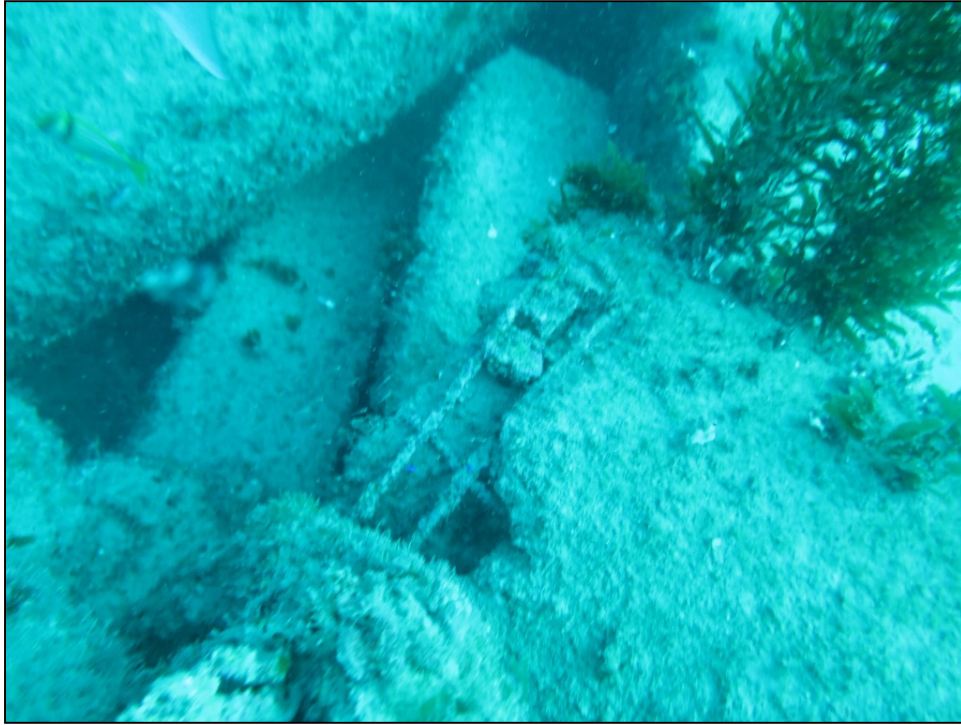
Photograph 2. Damaged, corroded, and exposed rebar typical of many of the ends of the concrete culverts and poles on the South County Artificial Reef Site 14 showing growth.
