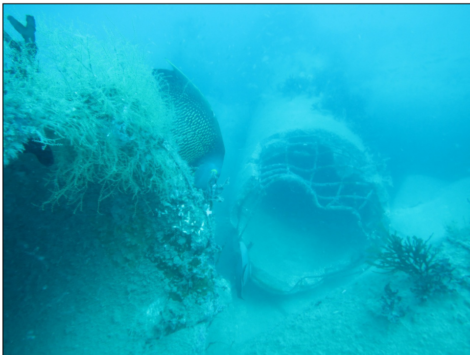
Photograph 2. Damage and exposed, corroded, rebar typical of many of the ends of the concrete culverts on poles on the Reef.
