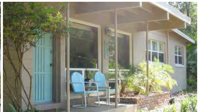
Pipe columns on a porch, Gainesville, FL
