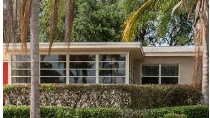
Large horizontal awning windows, Orlando, FL
